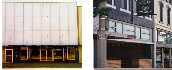
Before 120 N. Main Street After
