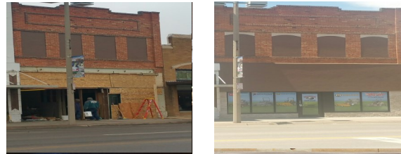
Before 309 N Main After
