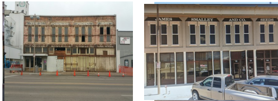
Before 322 N Main After
