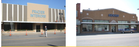
Before 311 N Main Street After
